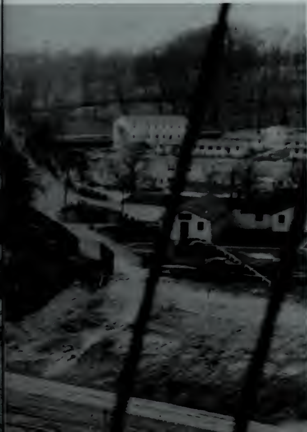
Early site preparation, Navy Annex in background
